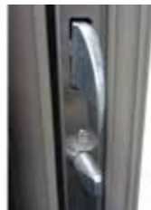
Multipoint 3 hook lock to opening door
